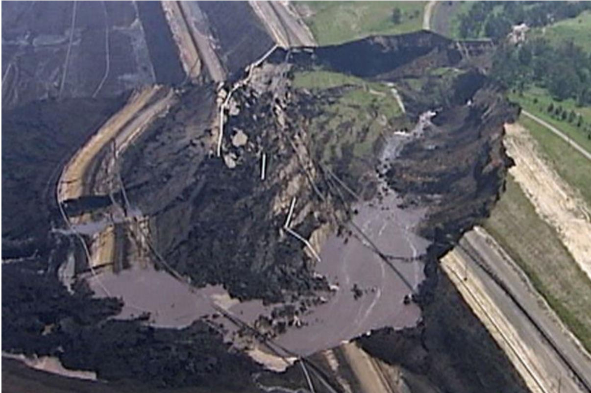
Aerial view of the damaged coal mine at the Yallourn Power Plant in eastern Victoria. (ABC-TV)
